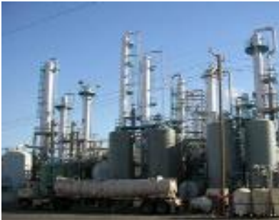
Romic plant on Bay Road in East Palo Alto
