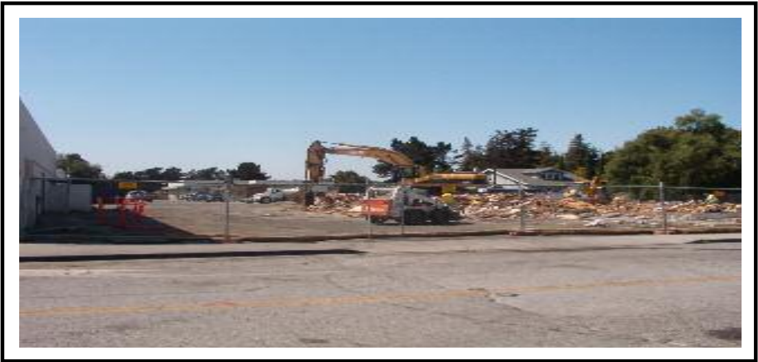
The demolition of the shopping area on University Avenue and Donohoe Street started at the end of September. The building of University Plaza is about to begin.
